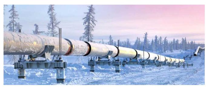
**Total length of Zapolarye-Purpe** is 488 km **Length of the aboveground section** is 320 km
