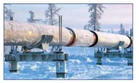
The Pipeline Supports Project for the main oil pipeline Zapolarye-Purpe. The above-ground method of laying in permafrost conditions was used for the first time. The contract amount – 14 bln rubles, over 20 000 supports, the time period – 1.5 years.
